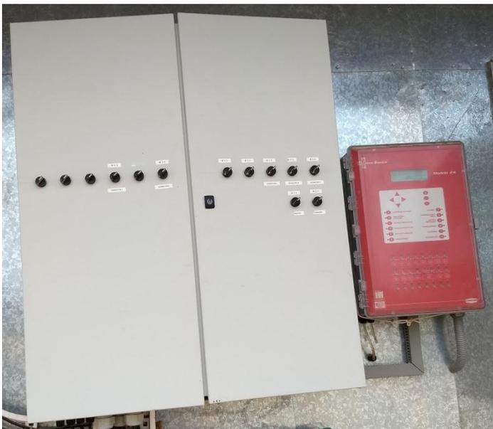
Figura 33 Tablero principal y Tablero de control Chore Tronics.
