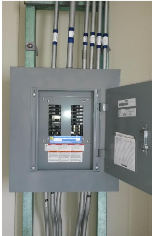
Fig. 3.2.4 Tablero NQOD304AB21S 3 FASES 4 HILOS
