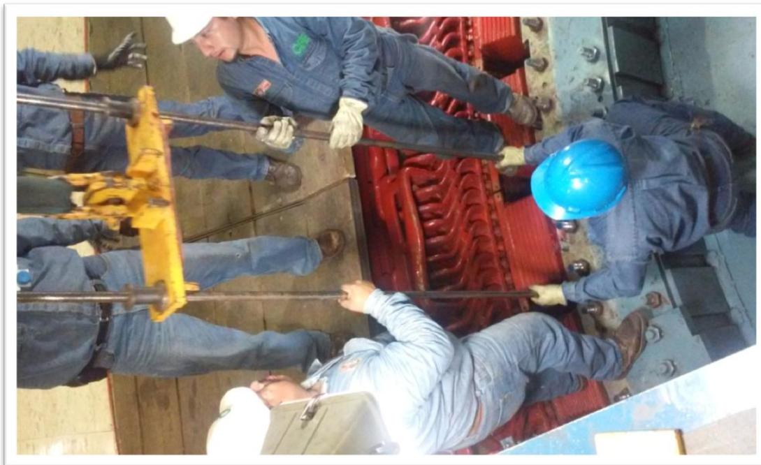
**FIG. C15** MONTAJE DE POLOS
