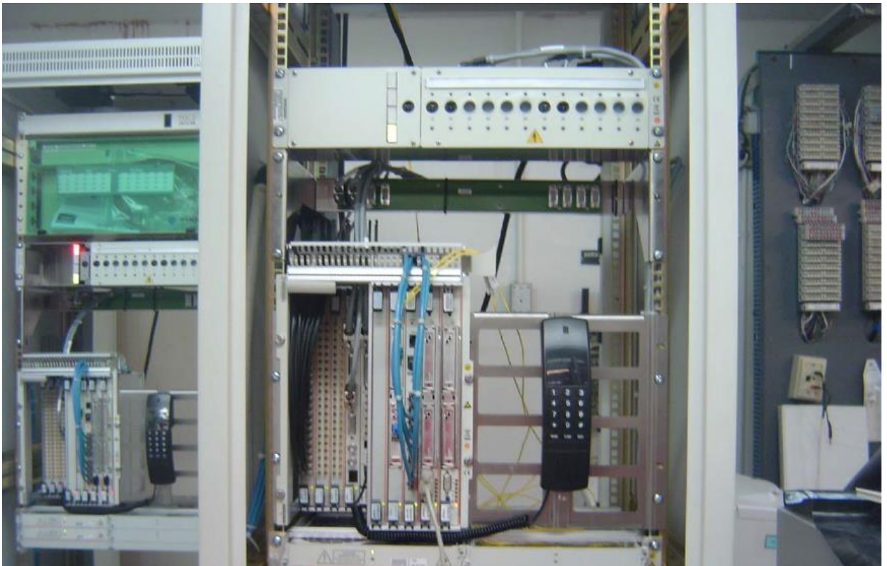
Fig.1 Nodo SDH Alcatel 1650SM-C
