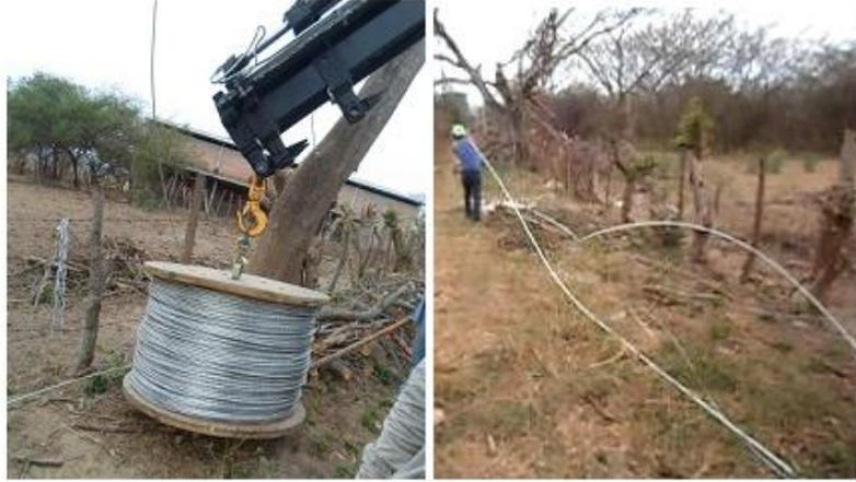
**Figura 3.24. Tendido del conductor 3/0**
